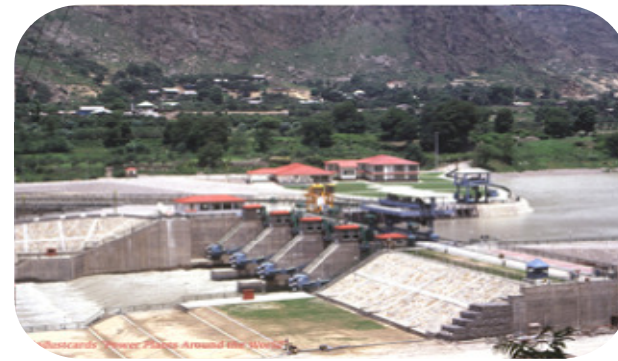
Jaypee Hydro Power Plant
